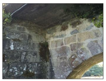
**Fig. 12:** Image captured with the quad copter drone, where you can see rooted vegetation in the joints of the ashlars and in the meeting edges (photograph by the author).
