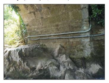
**Fig. 7:** Rocky substrate that serves as the foundation for the southern abutment of the Ponte Olveira Bridge (photo taken with the drone).
