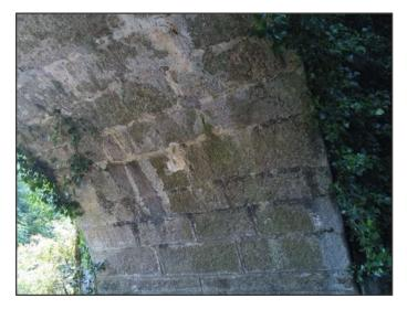
**Fig. 10:** Image captured with the quadcopter drone, where various lesions can be observed on the intrados of a vault, such as dark crusts or organic matter (photograph by the author).
