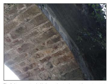
**Fig. 9:** Image captured with the quadcopter drone at the western start of the vault, where various injuries can be seen, such as dark scabs (photograph by the author).
