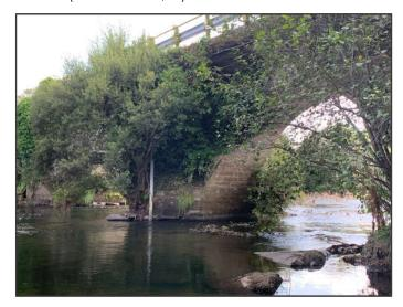
**Fig. 3:** Intermediate arch vault of the Ponte Olveira Bridge with abundant vegetation on the cutwaters, in a photograph taken by the drone (photo by the author).
