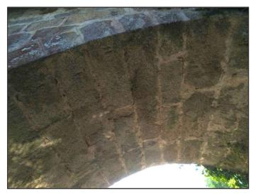
Fig. 11: Image captured with the quadcopter drone in the upper part intrados of the second arch vault, where in addition to the previous injuries we can see mortar deterioration (photograph by the author).
