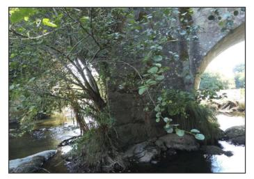
Fig. 13: Image captured with the quadcopter drone, where we can see abundant vegetation rooted on the firstpier (photograph by the author).
