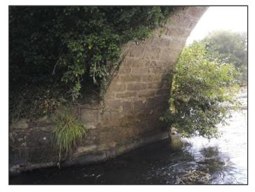
Fig. 8: Start of the third pier (counting from the south bridge abutment), and its corresponding cutwater, on the Ponte Olveira bridge (photo taken with the drone).
