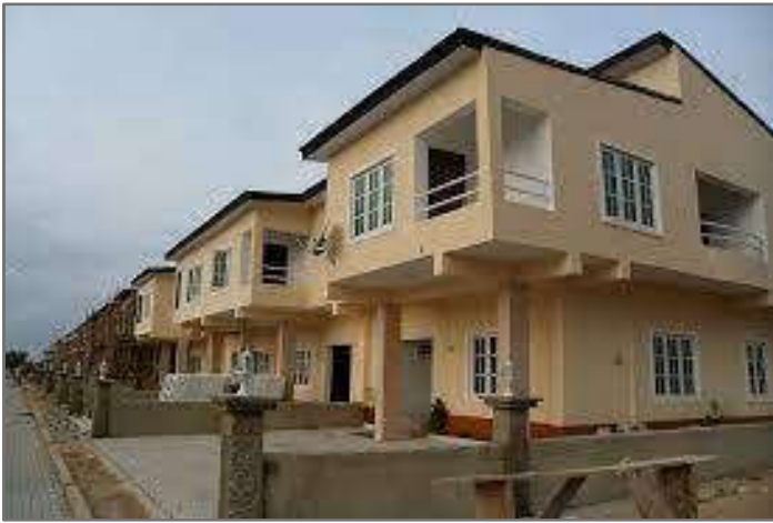
Figure 1: Lekki Gardens Eco-Estate, Lekki, Lagos, Nigeria.
