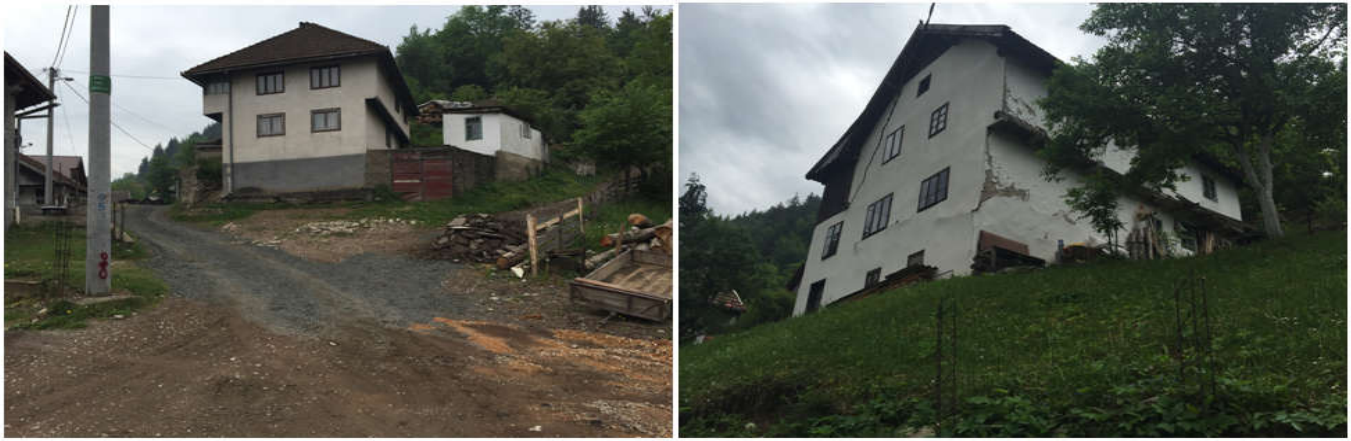
Figure 16. Reconstructed and renovated house built before World War II Source: Author (2020)
