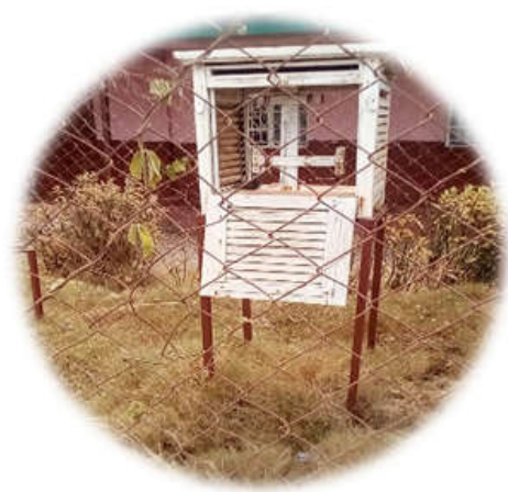
FIGURE 2: Abandon & dilapidated Meteorological Station at AMSSK
